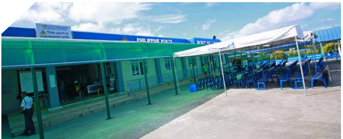
Below: The newly-renovated PTB in the Port of Lucena
