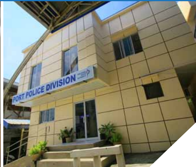
Above: The newly constructed Port Police building in the Port of Dapitan is equipped with surveillance room and newly-installed high-definition CCTV cameras for security monitoring within the port premises.
