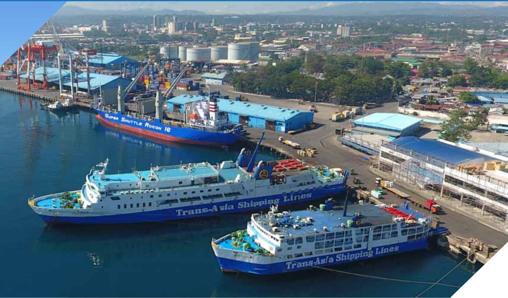
Above: The Port of Cagayan de Oro, one of the country's most bustling ports, services international cargo and passenger vessels routinely. The new Passenger Terminal Building (PTB) being constructed across the wharf is set to open in July 2019.
