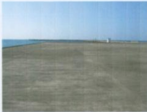
Concrete Back-up Area Area = 3,840 sq. m. (Port of Curimao, Ilocos Norte)
