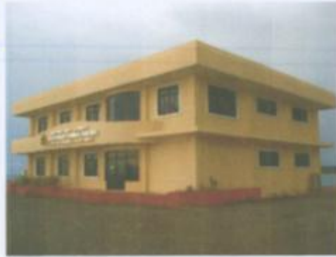
Two-Storey PTB (Port of Curimao, Ilocos Norte) Area = 300 sq. m. (1 st floor only)
