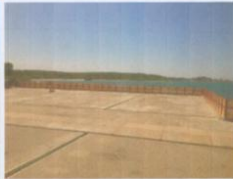
Concrete Back-up Area Area = 10,000 sq. m. (Port of Curimao, Ilocos Norte)
